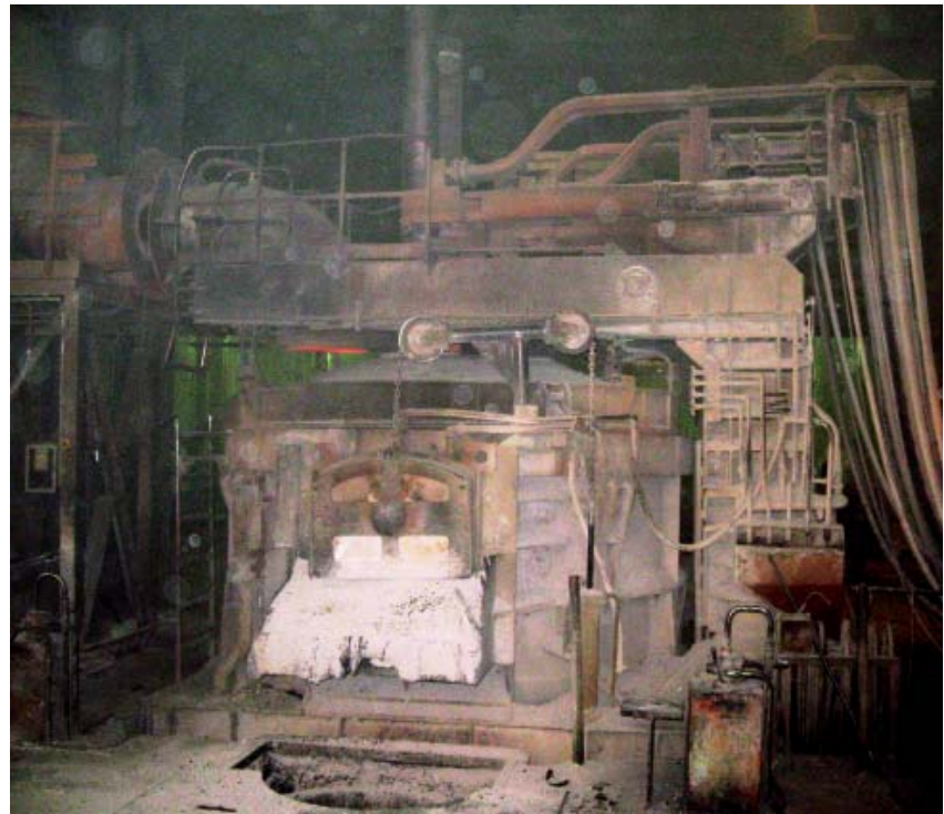
Figure 1: Electric arc furnace 1 before the overhaul.
